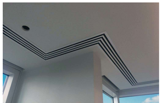
Colman CES Slot Diffuser complete with mitred corner sections installed at Bank of New York, London.
